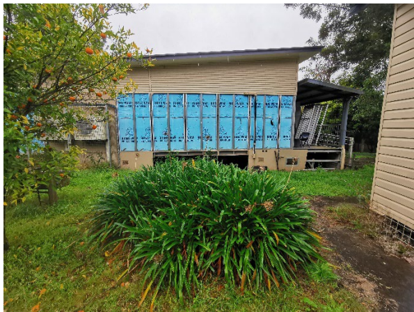
Photograph 3: Orchard area within the central northern portion of the site and adjacent unoccupied buildings.
