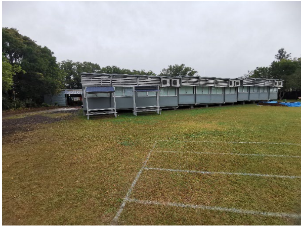
Photograph 1: Temporary demountable building on site
